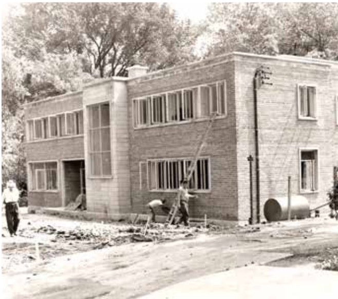
Workers put finishing touches on the building in 1957
